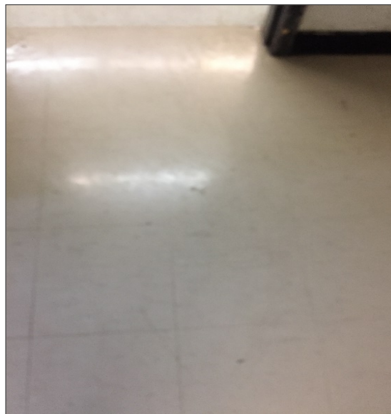
Photograph No. 17: Non-asbestos vinyl floor tiles within the corridors Loc.'s 52 and 58 (Samples 0038A-C).
