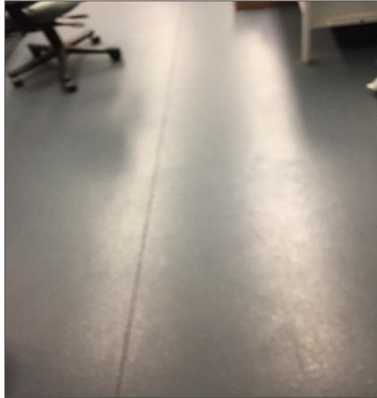
Photograph No. 8: Non-asbestos vinyl sheet flooring within the pool entrance Loc.39 (Rubber).
